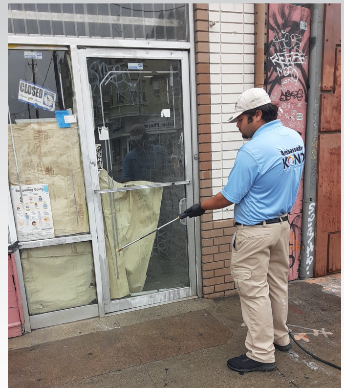
Fernando O., Graffiti removal with pressure washer
